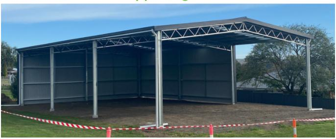
The tradies have been very busy over the last couple of weeks! Our Covered Outdoor Learning Area has been constructed, and plumbers have been busy this week connecting stormwater drainage. We are hopeful that this project will be fully completed over the next 4-6 weeks, with earthworks, concreting and the laying of synthetic turf still to take place.
